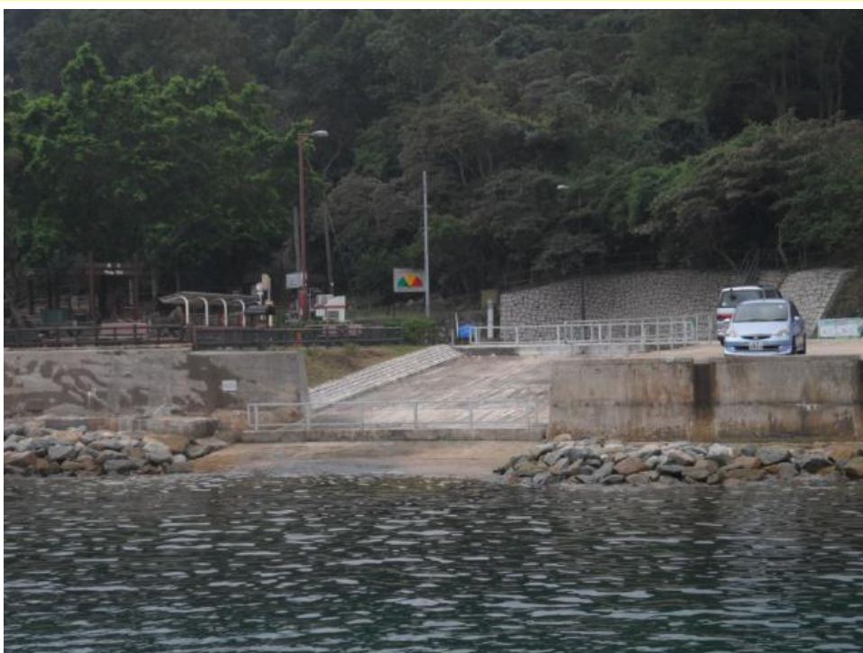
Example: Wong Shek Slipway
