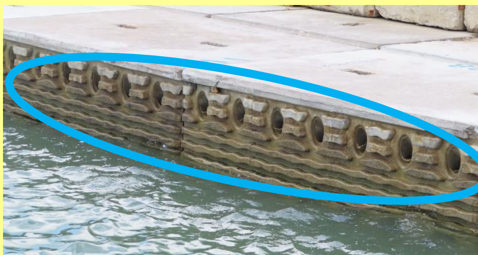
Example: Vertical Eco-shoreline at Tung Chung (eco-tiles)
