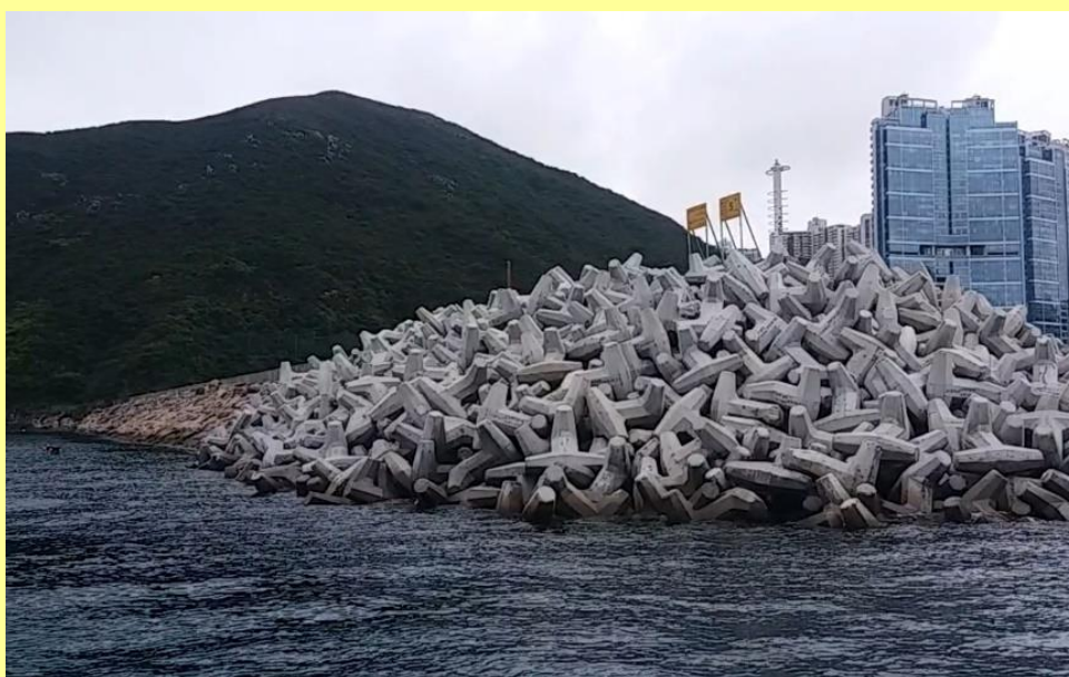
Example: Precast wave breaking units
